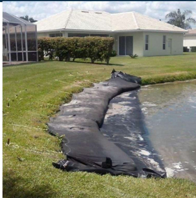
Filling GeoSOX with Sediment
