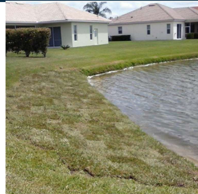
Sodding Over GeoSOX
