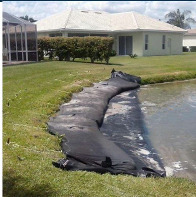
Filling GeoSOX with Sediment
